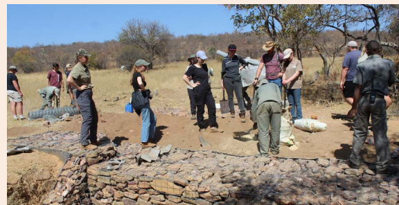
Students learned how to construct effective gabions in gull-eroded areas.
